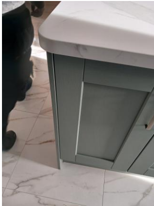
Photo 18B Kitchen island — second outer cabinet door with tight margin. 20260903_084145.jpg
